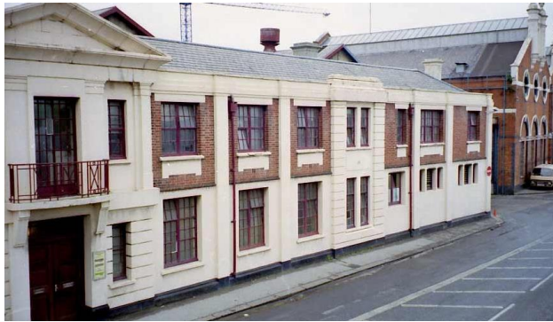
Recording of Reading Transport Office Block in Mill Lane
