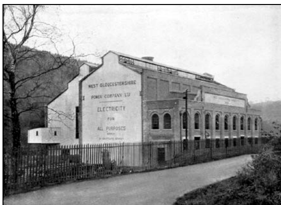
Lydney Power Station
