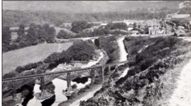
The timber viaduct that carried the tramway over the river to Torrington Station (on right)
