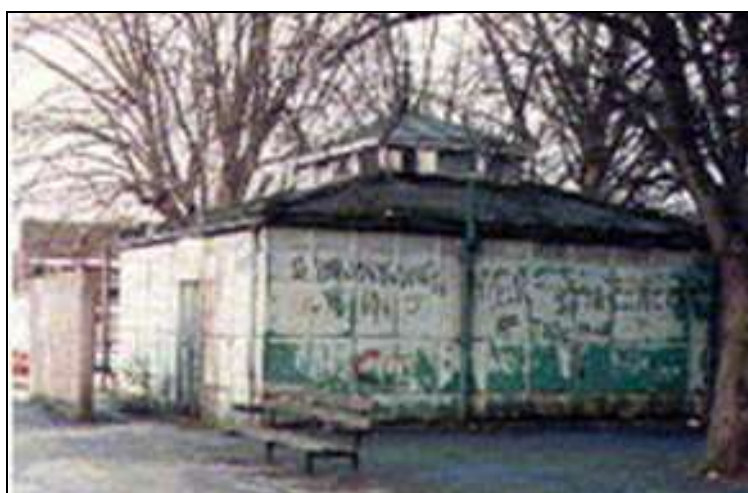
Caversham Road cast iron Public Convenience in original position
