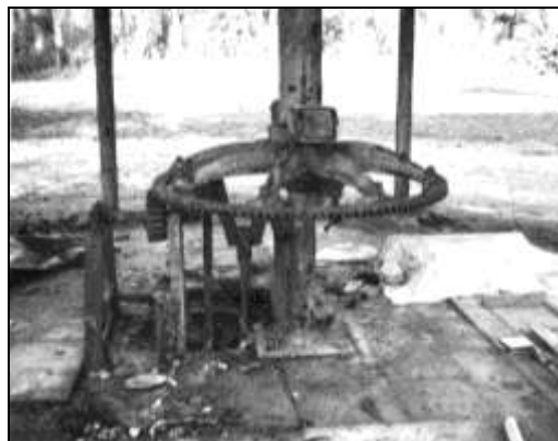
Horse wheel at Shabden Court showing pump gearing
