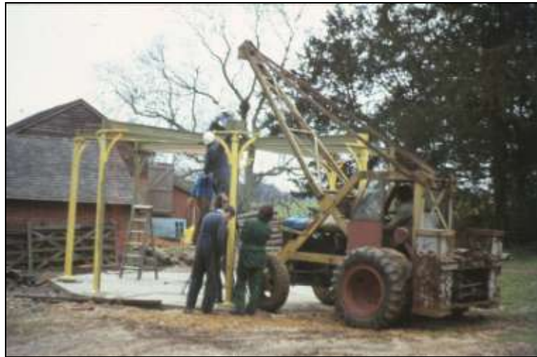
Horse Wheel at Greys Court (most of ironwork in position)
