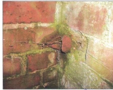
**Figure 4** The outlet pipe in close-up. This one is chipped but is thought to be near to its original length
