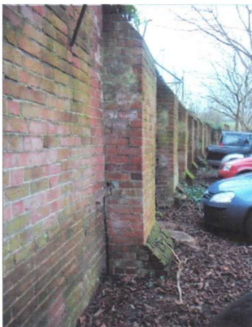
**Figure 1** One of the buttresses outside the wall, side outlet two thirds of the way down, hard against the wall. The lower courses are not keyed into the wall.
