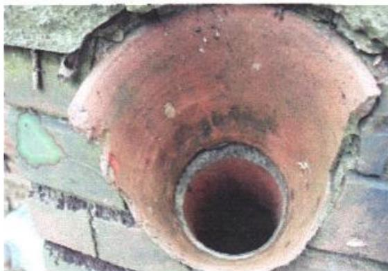
**Figure 2** The top of a pipe, rim broken, showing its 'flowerpot' shape and its junction with the glazed down pipe.
